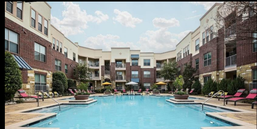
EMIF II, The BLVD, Irving, TX
